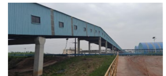
Fully Enclosed Belt Conveyor Corridors
