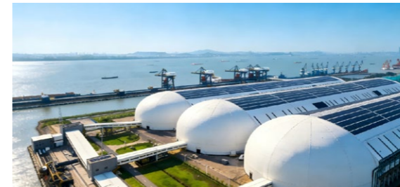
Distributed Photovoltaic System at Jiangsu Jingjiang Port Park
