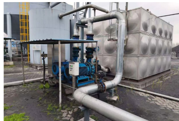
Nanjing Xiba Stockyard Triangle Area Reservoir Renovation
