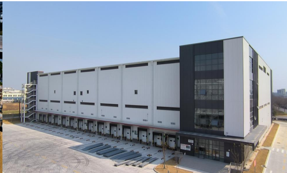
Nanjing Jiangning Project
