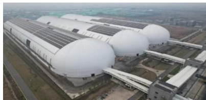
The Jingjiang Port shed has been covered with photovoltaic panels
