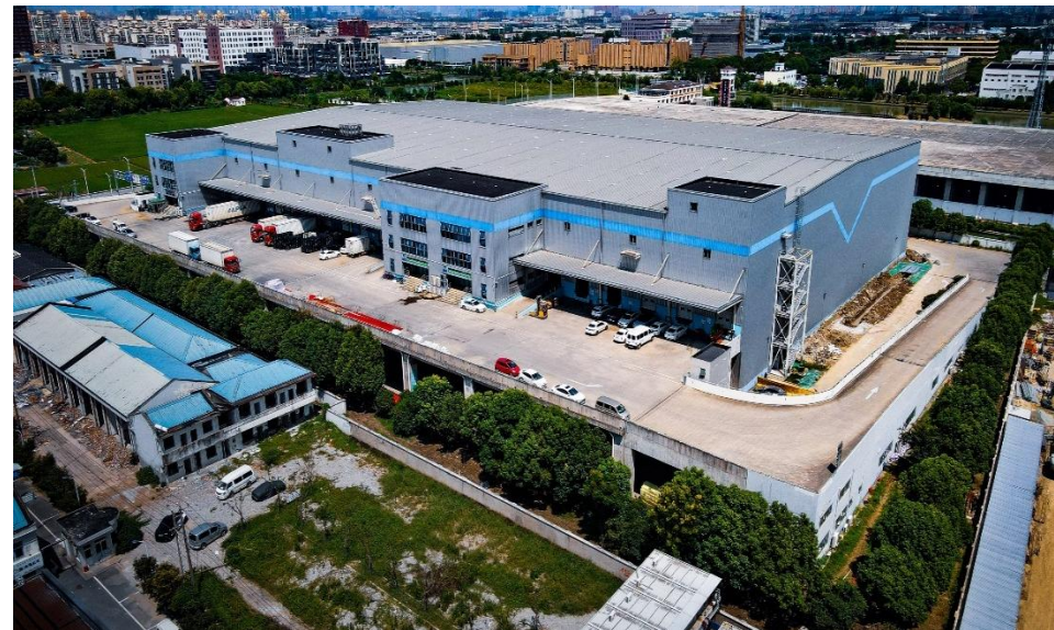
Shanghai Minhang Project (cold storage warehouse area of approx. 52K sqm)
