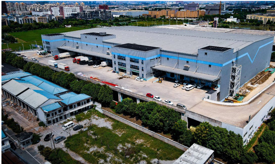
Shanghai Minhang Project (cold storage warehouse of 52K sqm) The transformation from a dry warehouse into a cold storage warehouse was completed and commenced operations at the end of 2023
