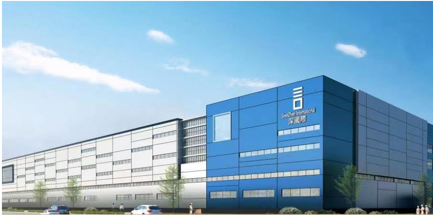
Chengdu Qingbaijiang Cold Storage Warehouse Project (completed and put into operation )
