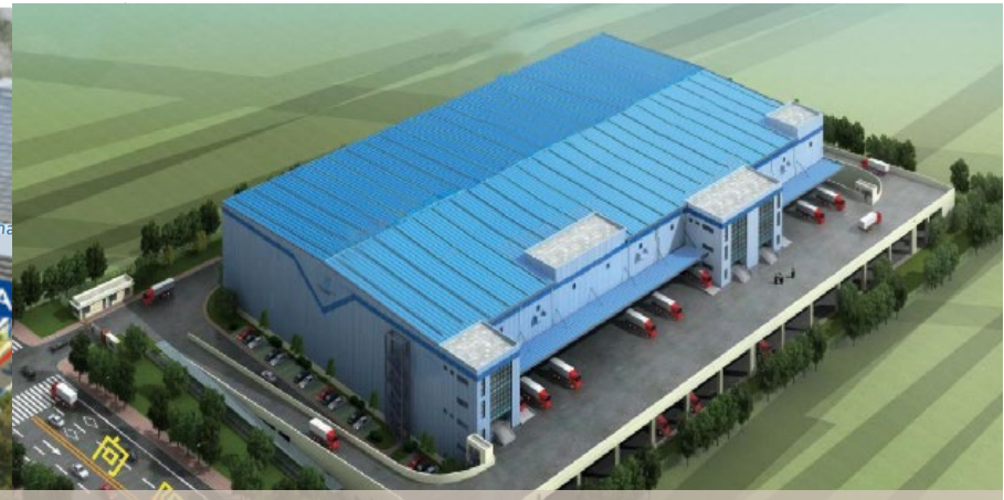
Shanghai Minghang Cold Storage Warehouse Project (completed and put into operation )
