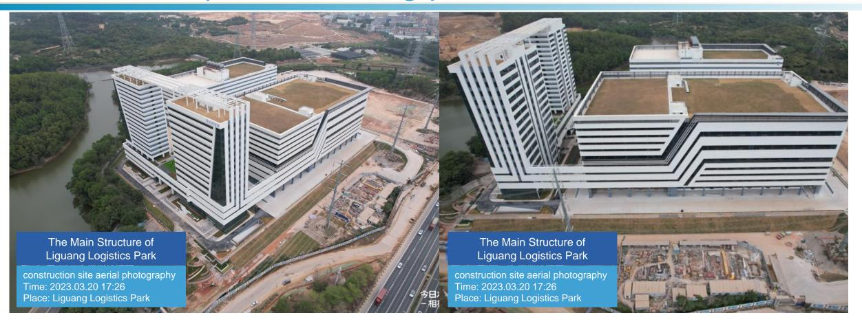
Site area of approx. 45K sqm; planned GFA of approx. 265K sqm. This project is designed to be a modern high-standard, intelligent and eco-friendly modern logistics park that sets an industry benchmark. The construction of the main structures thereof was completed with the roof completed in August 2022 and it is expected to be put into operation in 2023.
